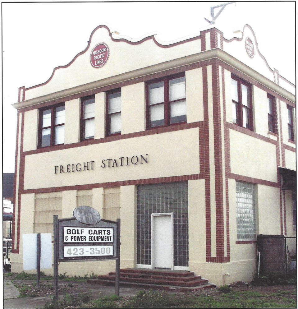
Former public entry on Harrison Street, north end of building, tracks to the right. Ron Goldfeder photograph.
